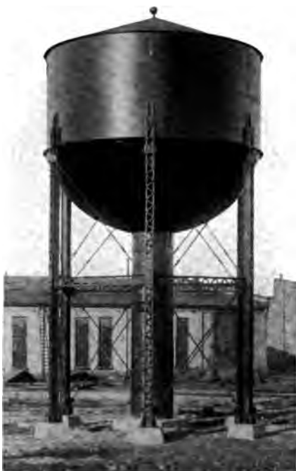
"Des Moines" Tank, 100,000 Gallons Capacity Built for Northern Pacific Ry. Co.
